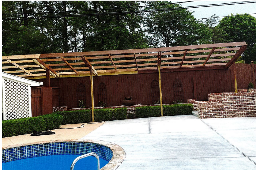
(Figure 2: existing sound mitigation canopy (view from the applicant's yard, looking north))
