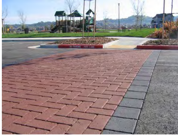
Stamped asphalt crosswalk
