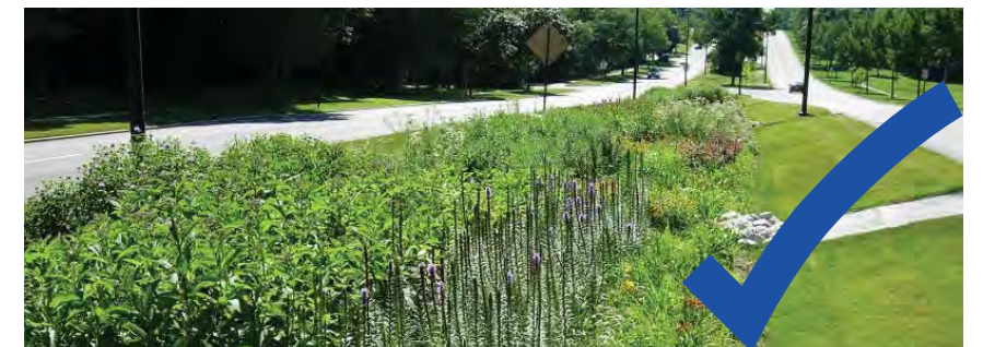
2. Bioretention Area Between Roadways
